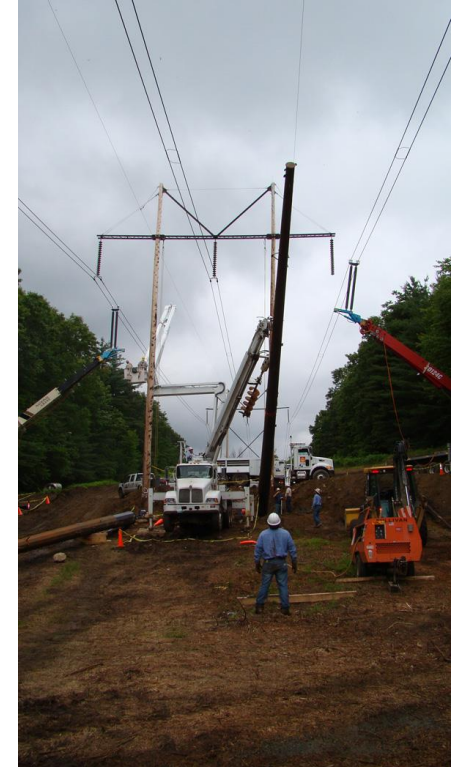
Example of wood structure replacement
