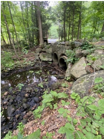
View S. downstream wingwalls & culverts undermined & separated from stone bridge.
