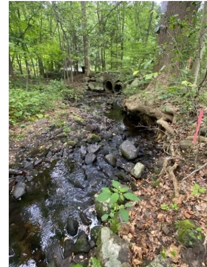
View S. downstream wingwalls & culverts undermined & separated from stone bridge.
