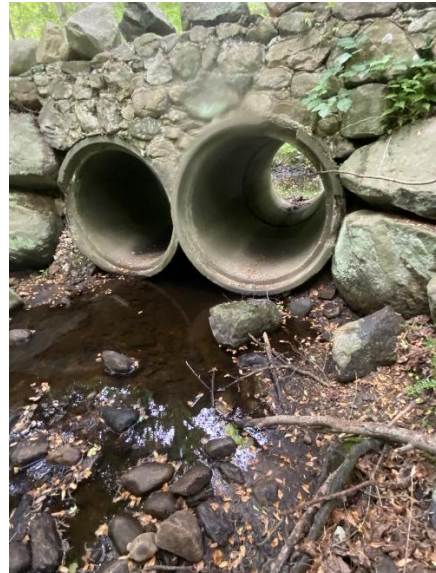
View N. Upstream two 60 in culverts upended w/o water flow.
