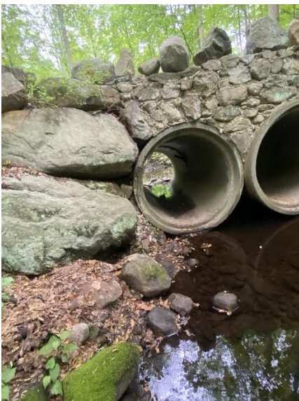
View N. Upstream two 60 in culverts upended w/o water flow.
