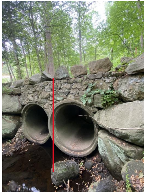
Culvert downstream edge damage. Ornamental boulders. No anchored rail. 7-8ft drop 90 Old Farm Site Development - Saini
