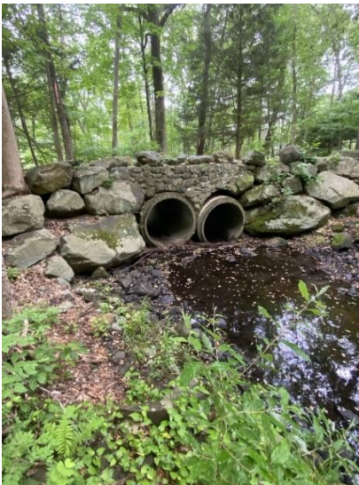
View S. downstream wingwalls & culverts undermined & separated from stone bridge.
