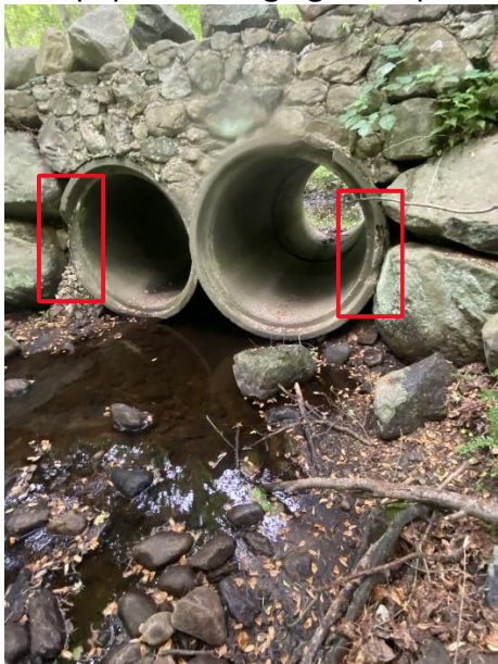
Culvert downstream edge damage. Ornamental boulders. No anchored rail. 7-8ft drop 90 Old Farm Site Development - Saini
