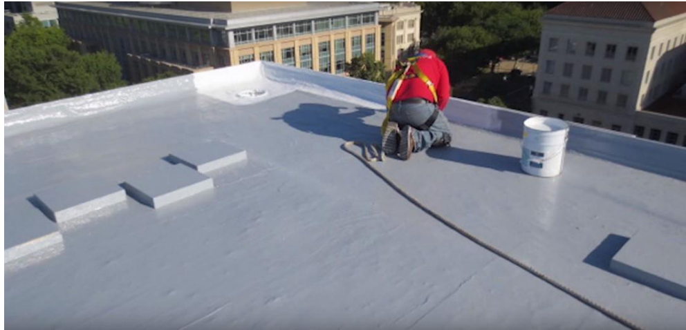
Photo by Reliable Roofing
