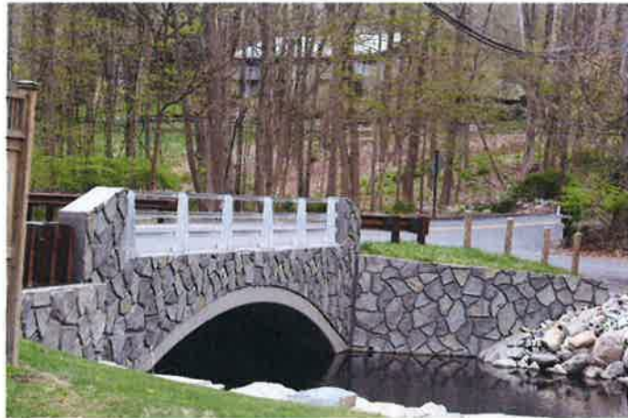
Cartridge Road Bridge
