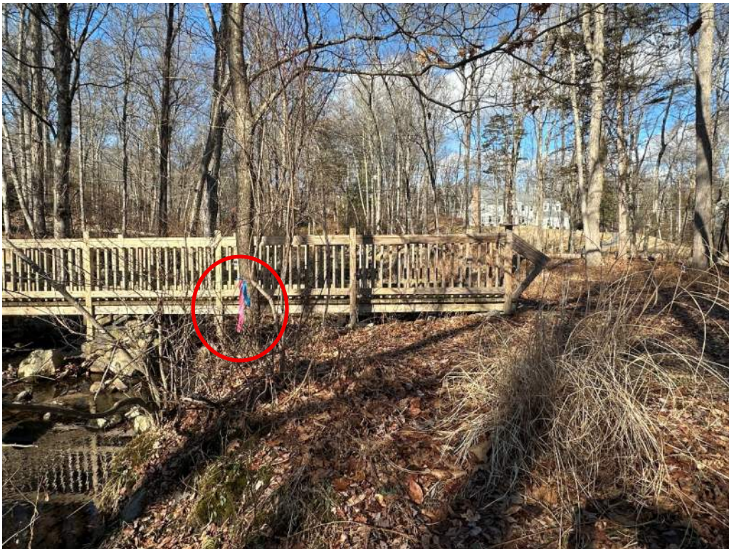
Photo 2: Wetlands Flags East End of Bridge (Looking North)
