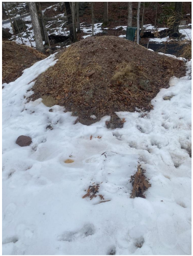
E. view close up of mixed fill construction debris pile
