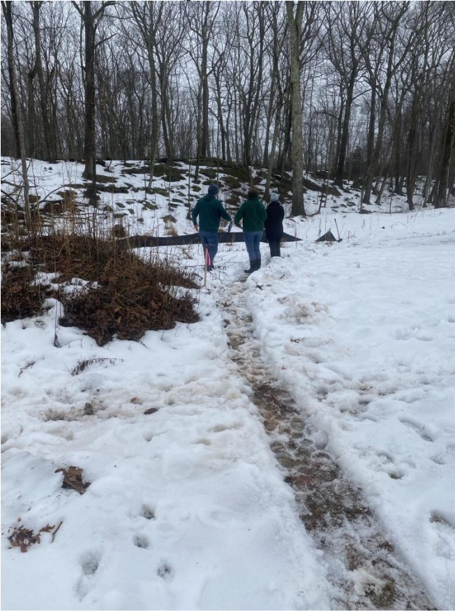
S. view beyond piles toward wetland and silt fence
