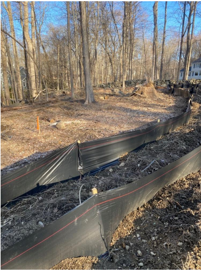
NW view silt line protects downhill cleared area
