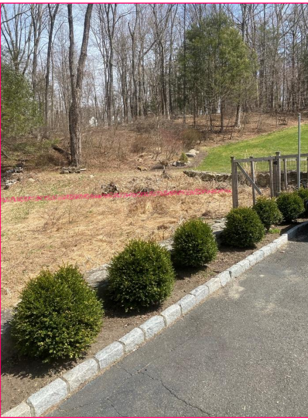
Silt fence to divert hillside flow away from job site
